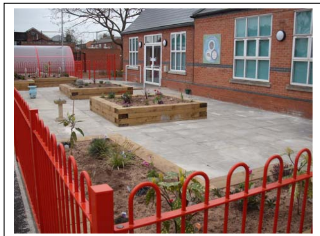
The new space complete with paving and raised beds
